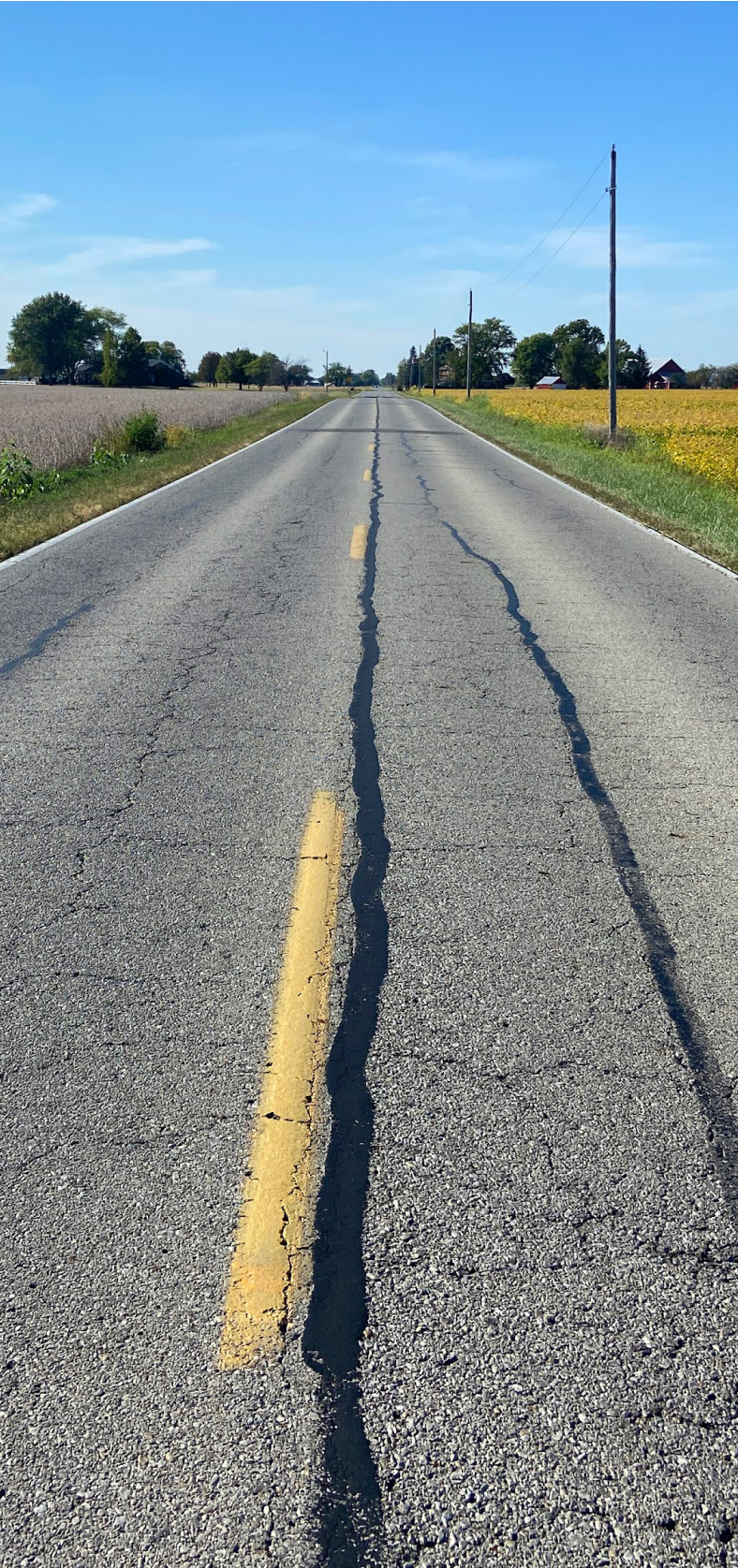
Rural Road in Madison County Image Source: HWC Engineering
